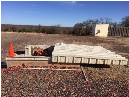
Trap house roof pulled all the way back
